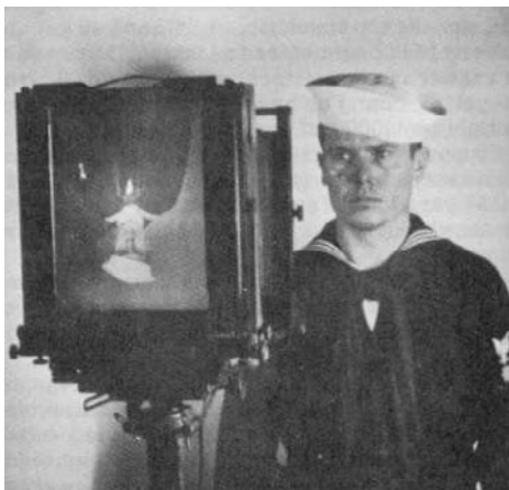
FIGURE 1.1: Image formation on the backplane of a photographic camera. Figure from US NAVY MANUAL OF BASIC OPTICS AND OPTICAL INSTRUMENTS, prepared by the Bureau of Naval Personnel, reprinted by Dover Publications, Inc. (1969).
